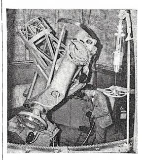
Operating in a manner similar to that of the original, a working model of the 200-inch astronomical reflecting telescope, which is being erected atop Mt. Palomar in California, was recently placed on exhibition at the 27th annual scientific display of the California Institute of Technology in Pasadena. The model, built to a 1/10th scale, is shown being examined by Dr. John Anderson, executive officer at Mt. Palomar Observatory.
