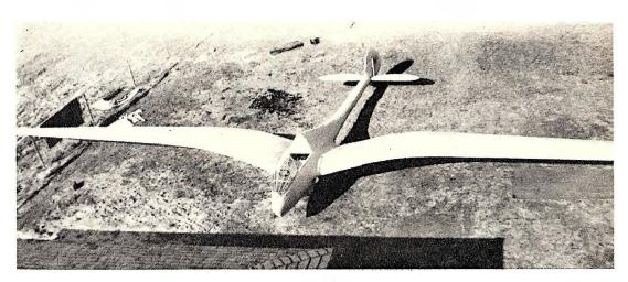
Featuring a full cantilever gull-type wing that gives it a truly bird-like appearance, a soaring glider constructed by Frank Merritt, of Glendale, Calif., has a wingspan of 72 feet and is believed to be the largest sailplane ever constructed in the
