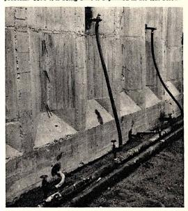
Above—Feeding cold water into the cooling pipes which are embedded in the dam's concrete walls at intervals of five feet.
