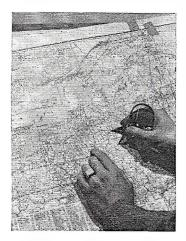
Designed to speed up and make the use of road maps more convenient, a new device combines a magnifier of high quality mounted in Zylonite, with a pair of hinged calipers for the estimation of distance between towns. The instrument is about two inches in diameter and comes in a neat leather pocket case. The colors are mottled black and white, green, and gray and red.
