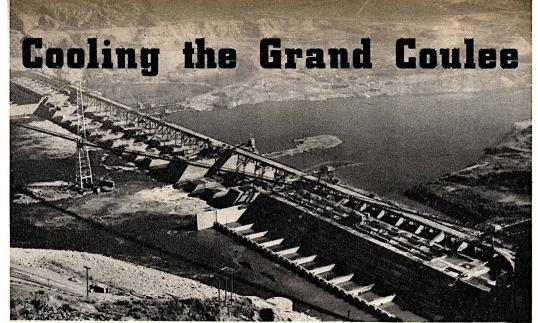
Grand Coulee Dam on the Columbia River in Washington (above) is about 50% completed. Cooling the tremendous heat liberated by the "curing" concrete is a major refrigeration problem. How it is being done is explained in the text below.
