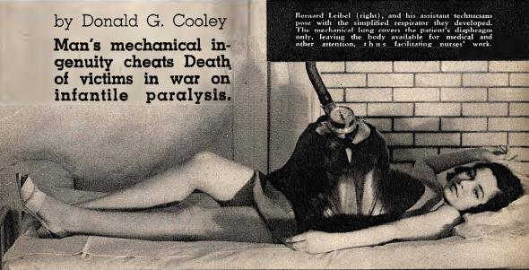
The compact rubber respirator shown above may soon replace the somewhat cumbersome metal chamber types. Like the larger "iron lungs" it creates a vacuum pressure that lifts and lowers the patient's chest walls, enabling breathing to be continued despite paralysed muscles. The aluminum framework is held to the patient's body by rubber fittings.
