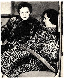
**DESIGNED** to hold passengers firmly in their seats in event of a crash so that they will not be thrown violently against the car interior, a newly developed safety belt for automobiles may eliminate injuries attributed to this cause.
