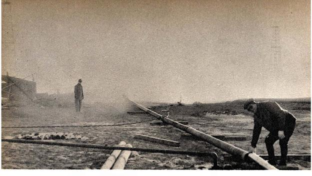
Lesh is shown placing nitroglycerin tubes in his pipe cannon. The torpedoes were drawn through the water cooled pipe and detonated at the mouth of the well.
