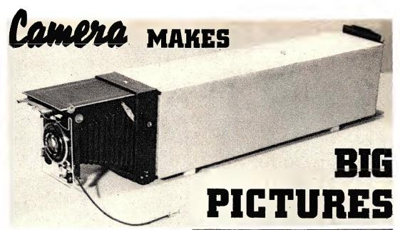
How the completed camera looks with the original camera on one end and the focusing panel at the other.
