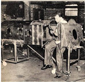
Shown above is a workman welding the air-tight chamber which is the essential part of an "iron lung" or disphragm respirator, as it is known professionally. A partial vacuum is produced in chamber when in use.
