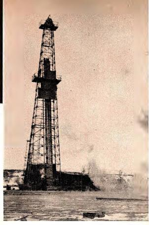
Everything was going fine. On down towards that oil sand at 4,100 feet went the bit. The continuous flow of mud, which picks up the drill cuttings and holds back the gas pressure, was circulating perfectly.
